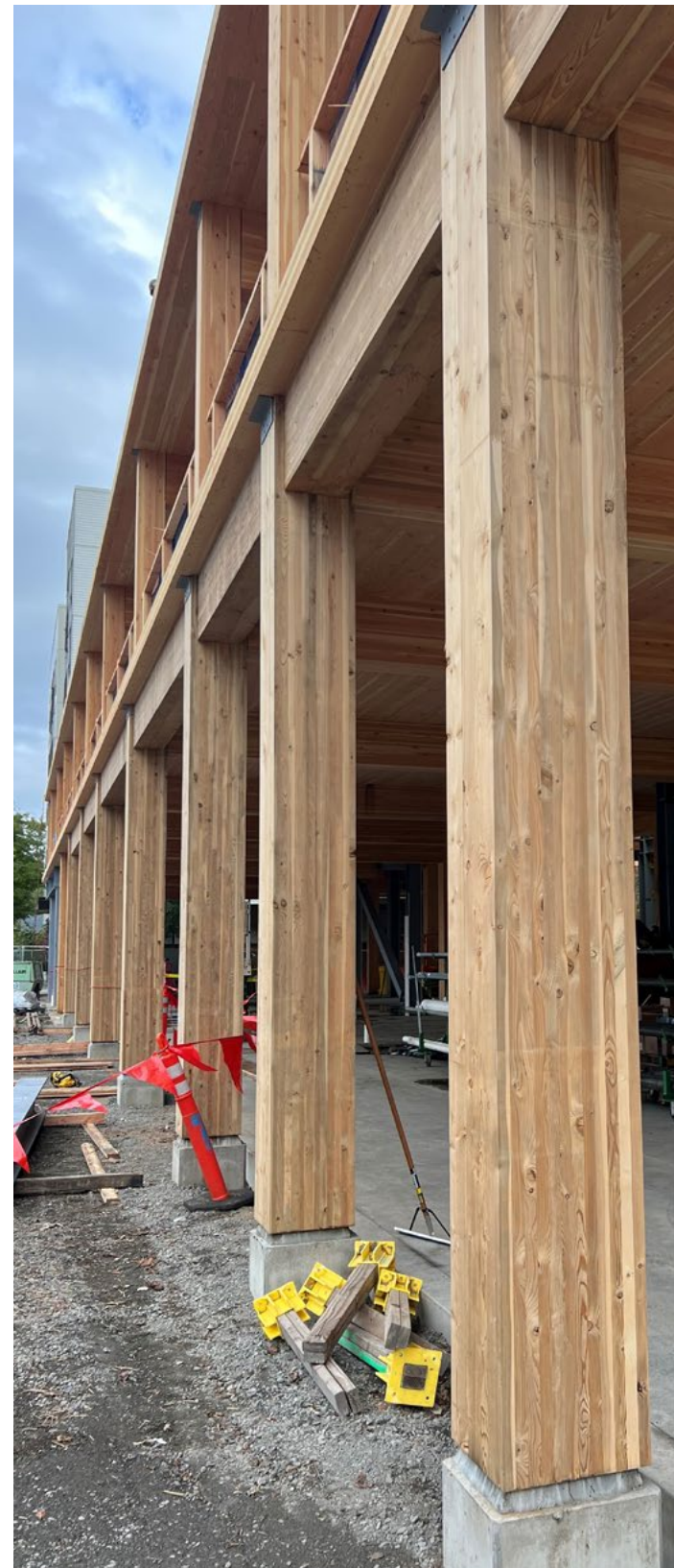
Exposed mass timber columns treated with Permapost KlearGard | 25™
