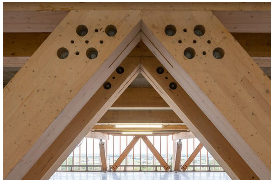
Silo by GRAAM, Dijon, France
